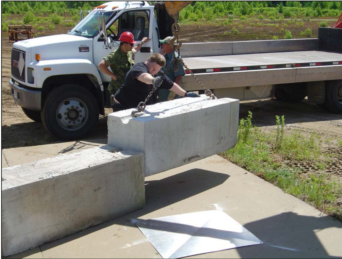
Figure 6-6. Installation of the concrete wall.
