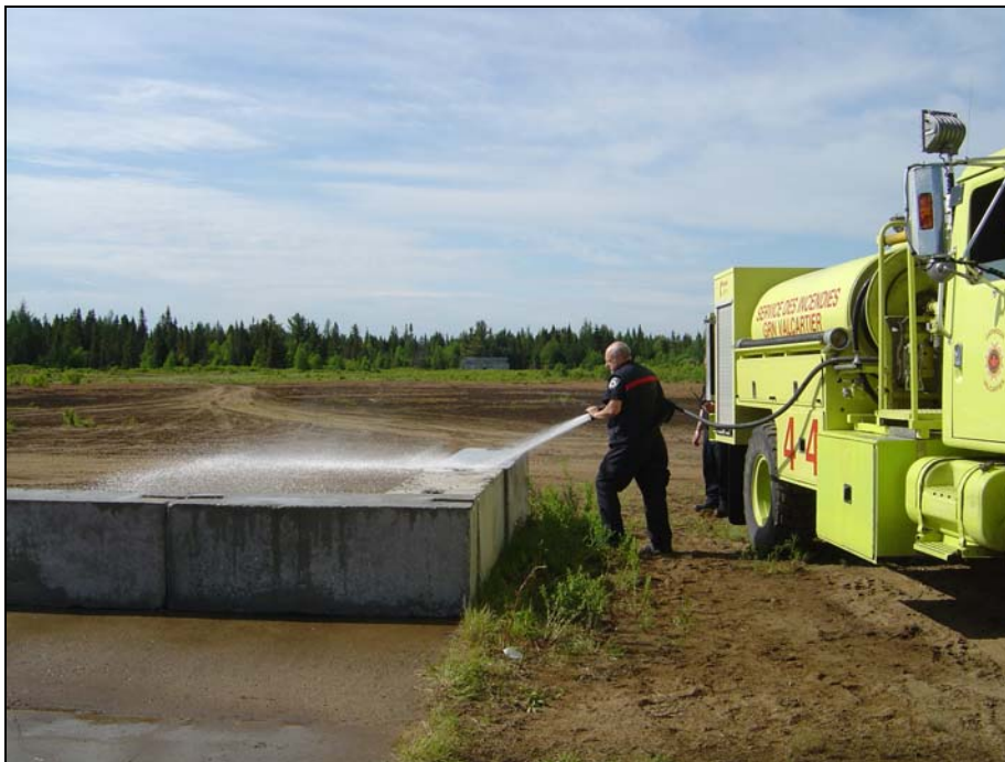
Figure 6-9. Washing the concrete surfaces.
