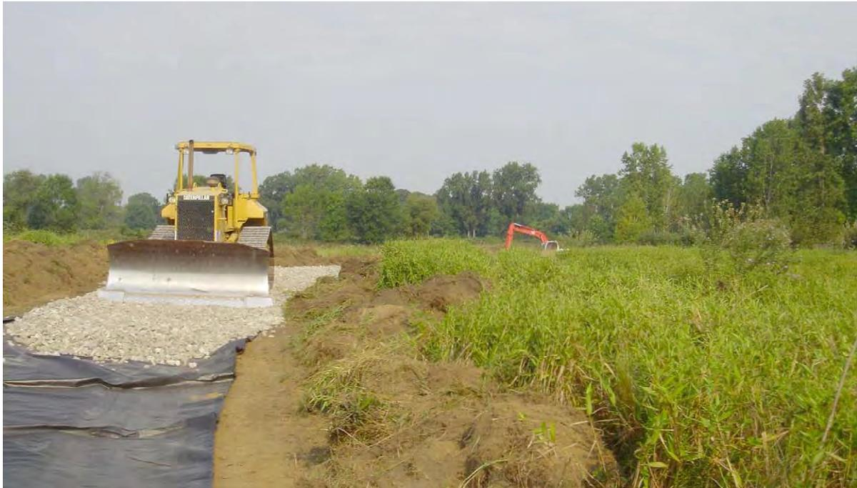
**Figure C-3. Construction of the paved road in PBOW.**
