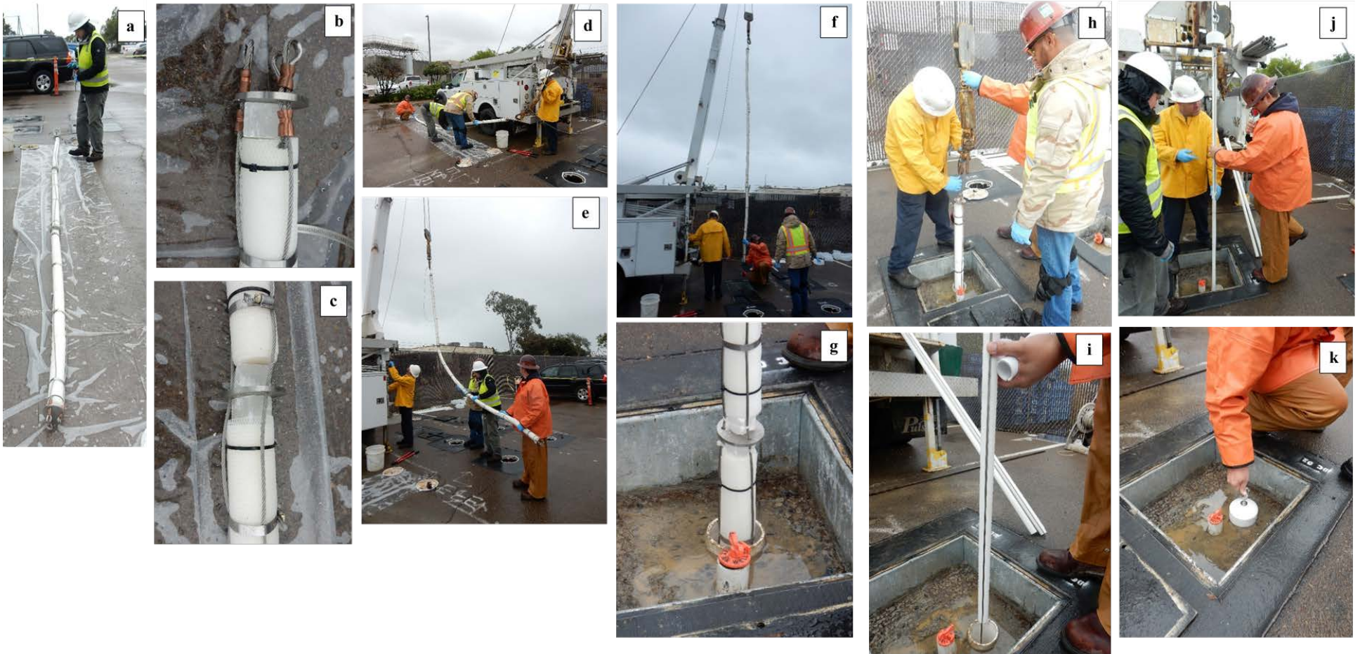
Figure 5.7. Cylinder Holder Design and Installation Showing 12 Cylinders Assembled in Holder (a), Close-up of Top of Holder Showing Stainless Steel Cables, Stainless Steel Alignment Disk, Wax Separator Block, and Plastic Cable Ties for Stainless Steel Securement (b), Interconnection Between Two Cylinders (c), raising the Holder Using a Drill Rig (d, e, f), Lowering into Well (g, h), Attachment of PVC Pipe with slit to Support Cable to Prevent Cylinder Floating (i, j), and Attachment of Well Cap (k).
